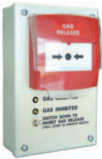
FP0570 Local Gas Control Station - Automatic. Local Gas Control Stations are used in gaseous fire extinguishing systems to provide local area manual control of a release. The automatic version includes a Gas Inhibit switch, buzzer and LED, whereas the manual version does not.
