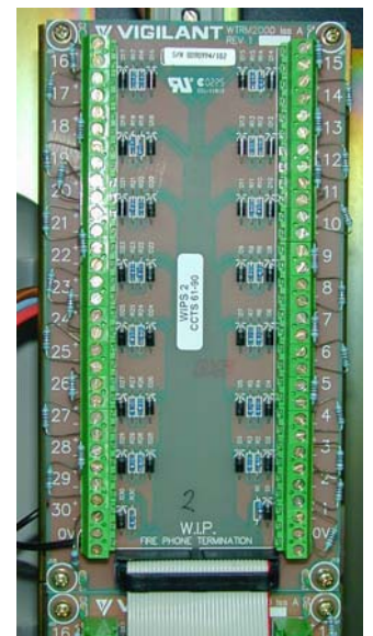
PA0916 WTRM2000 WIP Termination PCB
